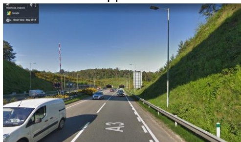
A3 Hindhead S approach to tunnel
