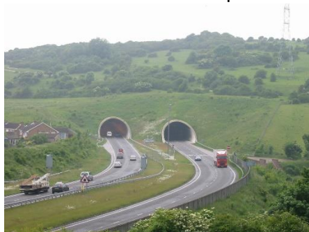
A27 Southwick Tunnel E portals
