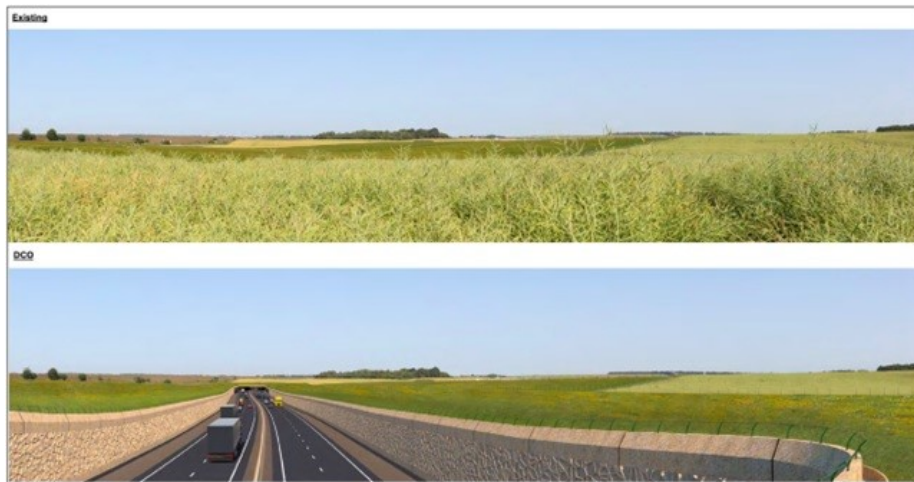
Cutting leading to western tunnel portal. Image by National Highways
