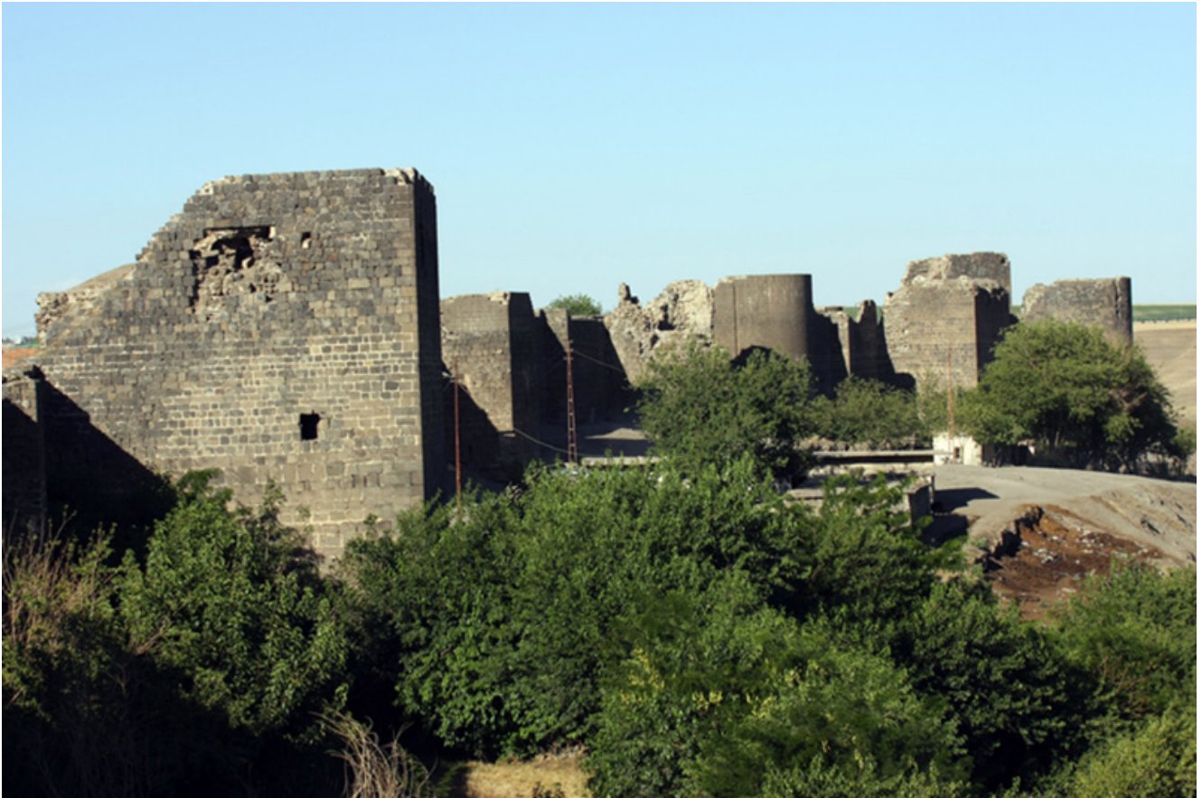
Diyarbakır Castle, Turkey, structurally damaged by earthquake © sadikgulec
