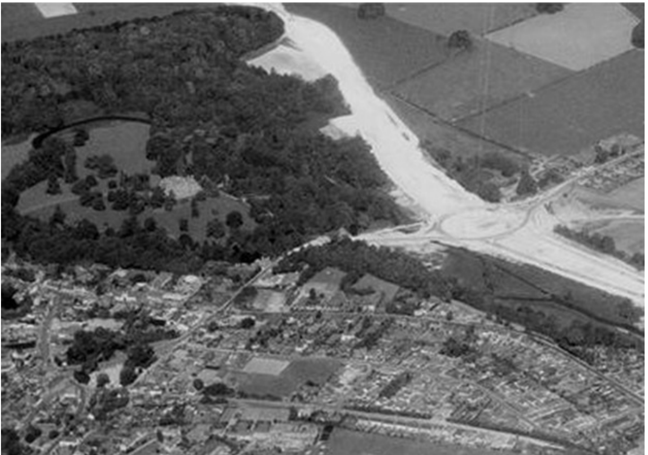
A303 Amesbury Bypass under construction 1968, showing the World Heritage Site landscape (designated 1986) deeply scoured
